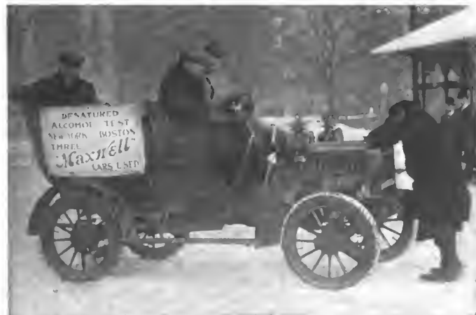
GETTING UNDER WAY FOR THE DAY'S WORK.
